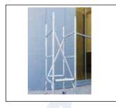
STEP-2 Fit diagonal brace from 1st rung to 3rd rung on sure diagonal brace to
