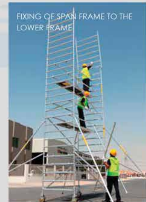
DOUBLE WIDTH 7 RUNG SPAN FRAME 6.5 Mtr. PLATFORM HEIGHT
